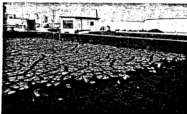
Once dry, the caked residue can be removed by mechanical loaders, a vacuum system or any number of other methods.
