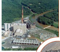
The CFB power plant in Seward, Penn. is the largest waste-coal plant in the world, and was built atop coal refuse and CFB asb.
